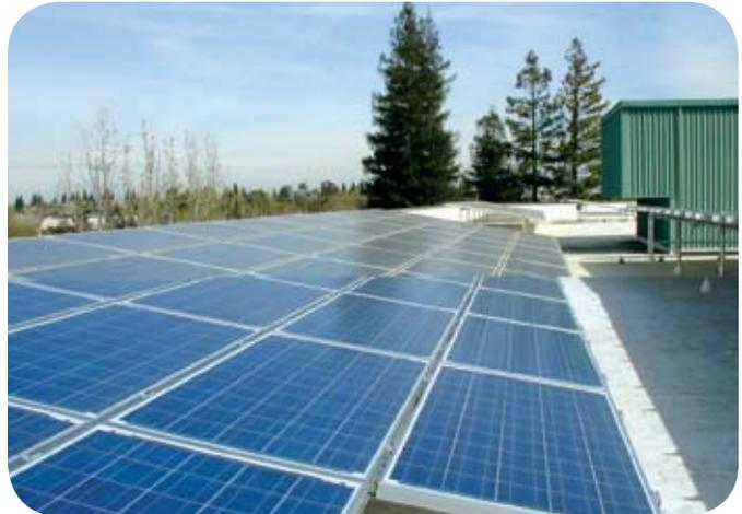
The county has partnered with SMUD to install solar panels on several buildings, including this 100 kW solar array for Sacramento County's Health & Human Services Building which came online in April 2008. In just 3 years, it has produced 450,000 kwh of electricity, reducing greenhouse gases equivalent to taking 61 cars off the road for a year. (Photo: Dan Mendonsa)
