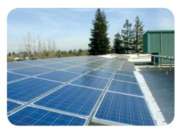
The county has partnered with SMUD to install solar panels on several buildings, including this 100 kW solar array for Sacramento County's Health & Human Services Building which came online in April 2008. In just 3 years, it has produced 450,000 kwh of electricity, reducing greenhouse gases equivalent to taking 61 cars off the road for a year. (Photo: Dan Mendonsa)
