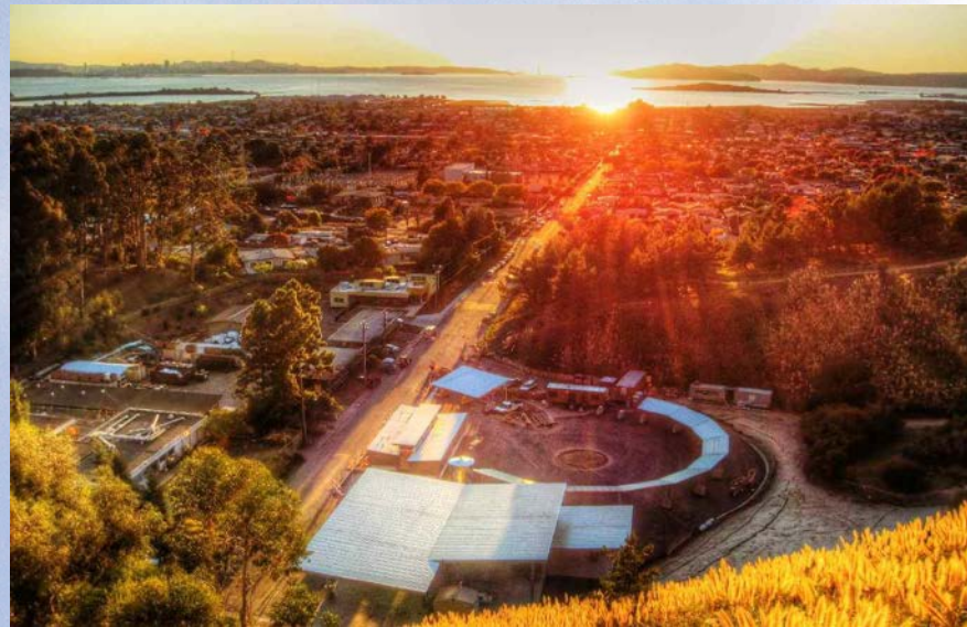
Construction of new LEED Platinum El Cerrito Recycling and Environmental Center
