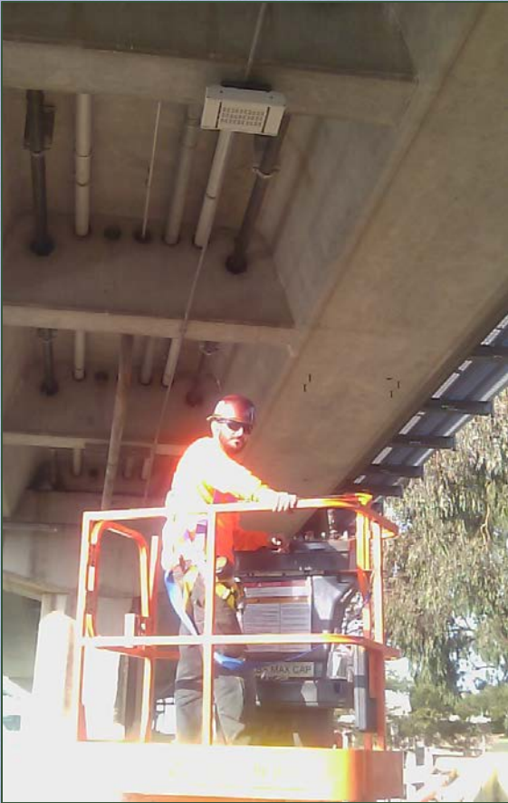
Ohlone Greenway LED Installation
