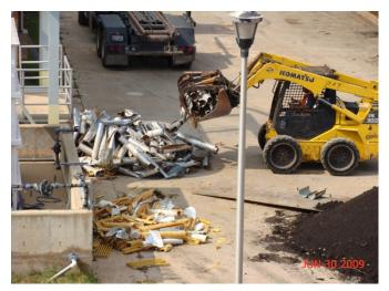
Figure 7.2. Recycling Aluminum Pipe Covers
