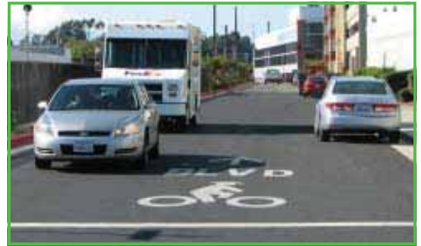
A large thermoplastic stencil with BLVD above a bicycle icon reminds motorists that they share this street with cyclists.
