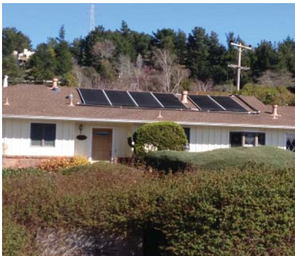
Home with solar hot water panels in Mill Valley
