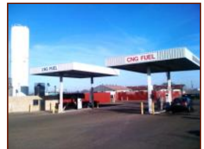
Tulare's CNG/LNG Fuel Station
