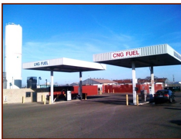
Tulare's CNG/LNG station
