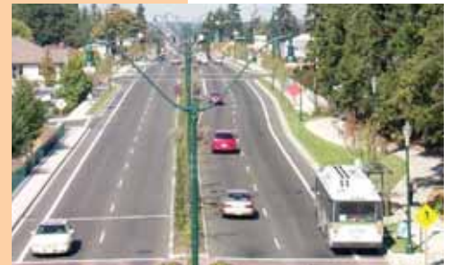
Bridgeport Way in University Place, WA before (above) and after (below) improvements were made.
