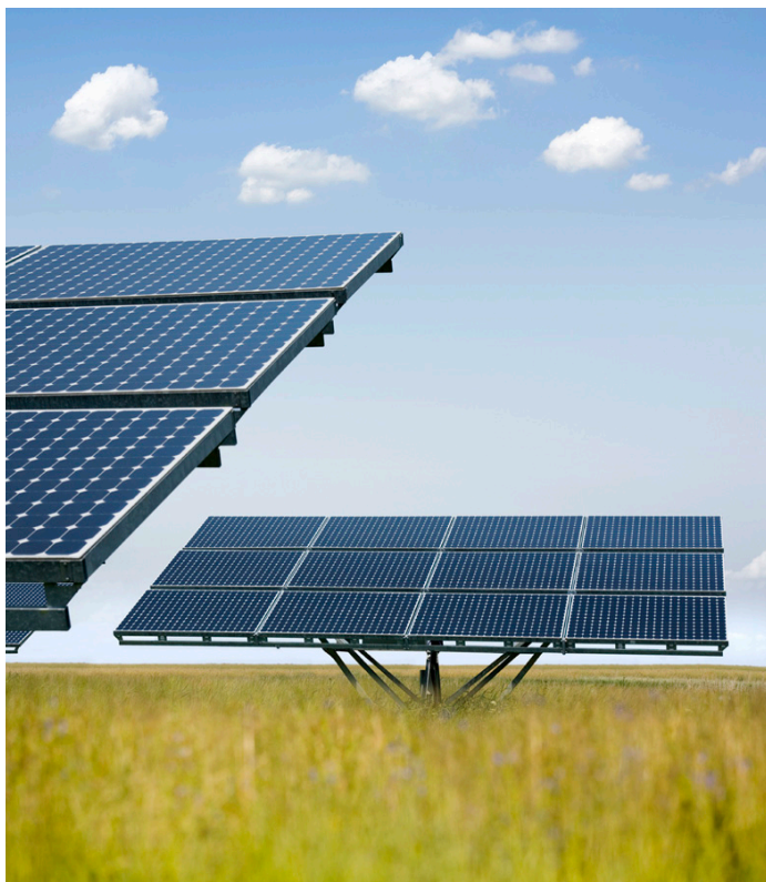
PV panels can help the City produce its own power.
