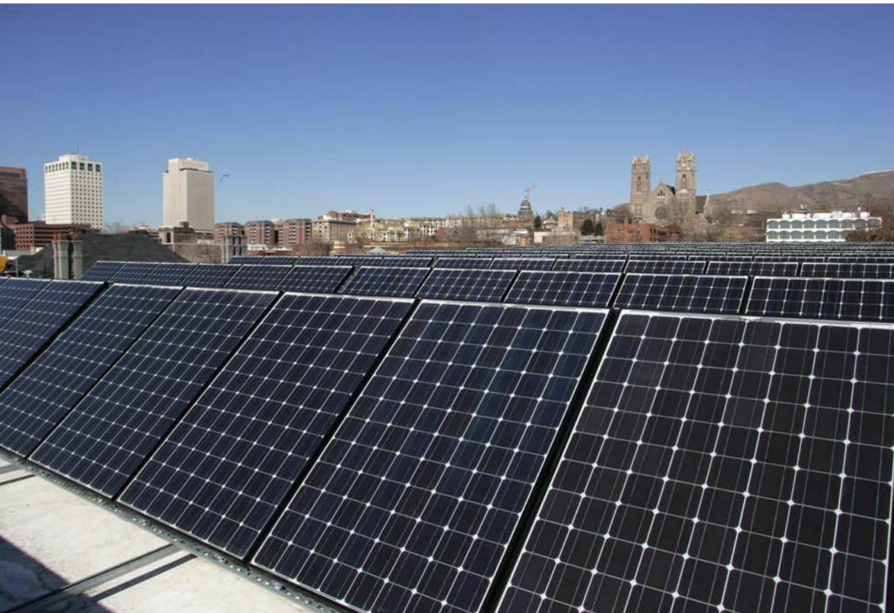
A 25-kW solar PV system provides power to the county-owned Clarke Planetarium in downtown Salt Lake City. (SLC/PIX18364)
