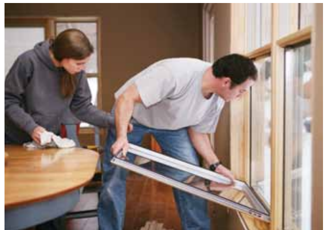
Retrofitting buildings with dual pane windows made with low-emittance (Low-E) glass reduces energy use.
