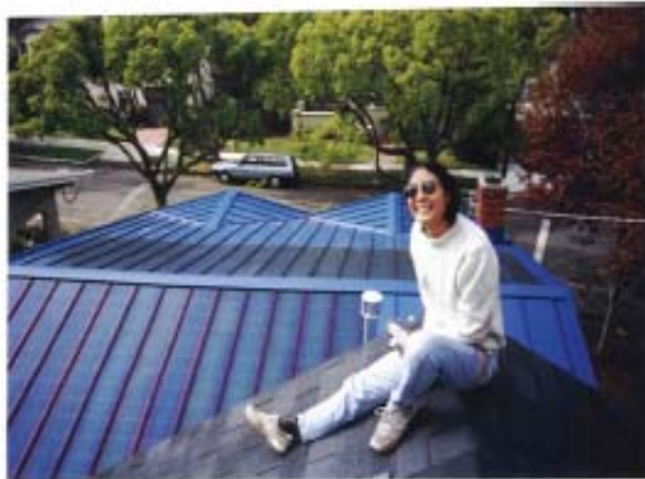
Standing seam metal roof
