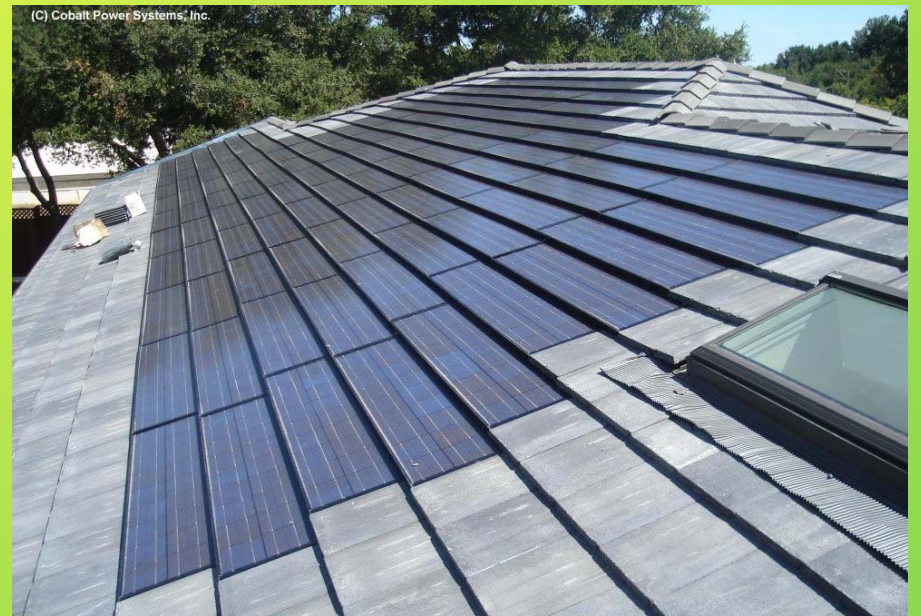
Sharp PV roof tiles
