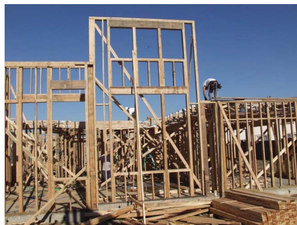
Building construction. Source: Union City.
