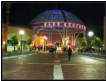
City Centre Cinemas, including retail and restaurants
