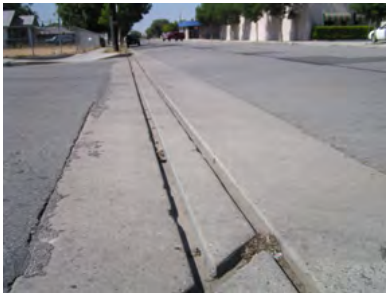
Bicycle unfriendly slot drain
