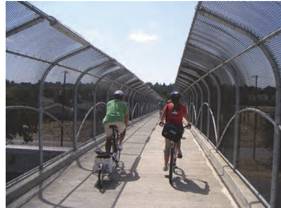
Crossing over an interstate in Davis, California
