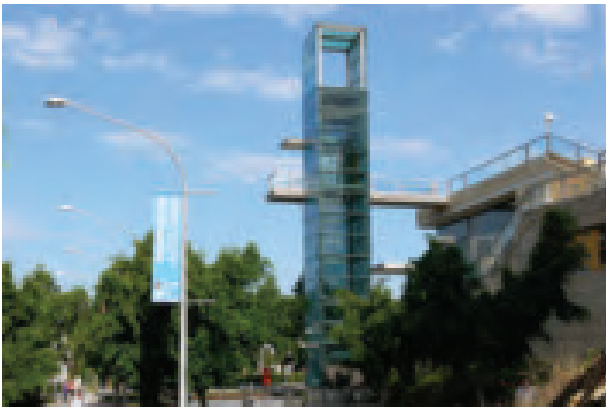
Public lifts with glass walls in visible places
