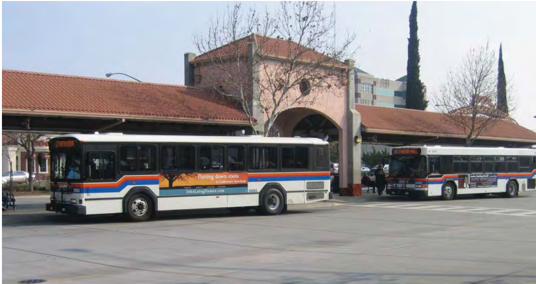
Bus Terminal, Modesto Centre Plaza, Modesto, California
