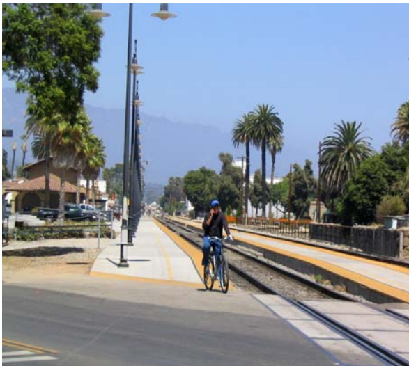
Photo 16a: this photo portrays the rubberized warning approaching the Railroad crossing.
