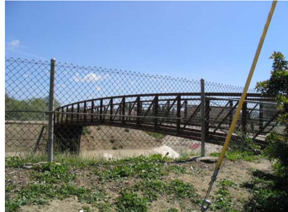
Photo 21: This bike/pedestrian bridge in the City of Lompoc successfully spans the missing link created by a flood plain. The bridge connects V St. to a Class I facility that runs to the east and is part of the regional bikeway network.
