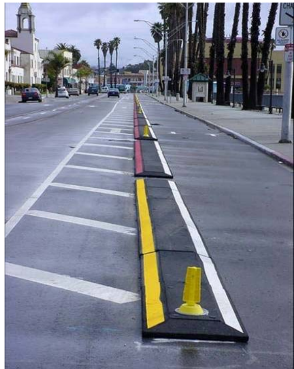
Photo 12: Contra-flow bike lanes in the City Cruz. Bicyclists can travel east or west on the section to the right. Photo courtesy of City of Santa Cruz.
