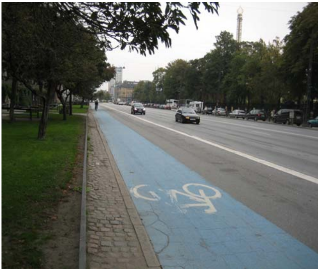
Photo 11: colored bike lanes in Copenhagen, Denmark are used to alert right turning motorists of their responsibility to yield to bicyclists at upcoming intersections.
