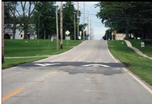
Figure 8. Driver view of speed table in Gilbert.
