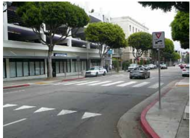
Advance stop bars and yield lines alert motorists of pedestrians and provide increased visibility for persons crossing the street
