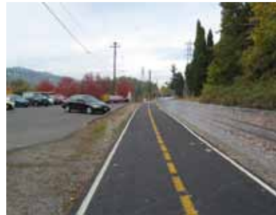
Open boundaries can be created where users may be entering the trail.
