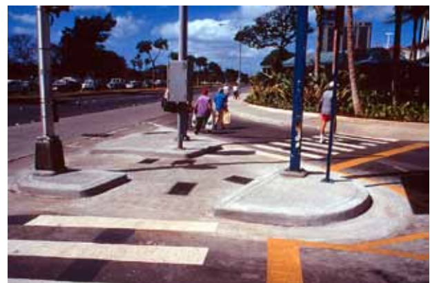
Pedestrian refuge islands break up a crossing and allow pedestrians to cross one side of a street at a time
