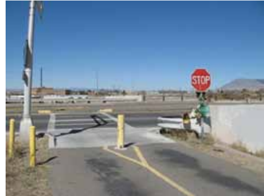
Bollards deter motorists from driving on the trail.
