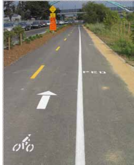
Centerline striping and directional arrows encourage trail users to provide space for other users to pass.
