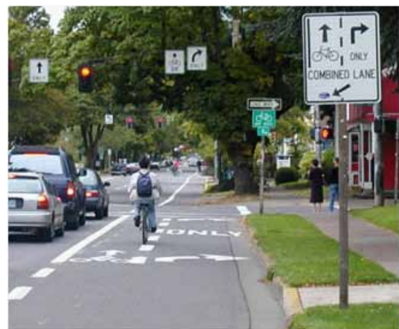
Shared bike-right turn lanes require warning signage as well as pavement markings.
