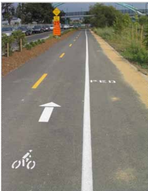
Class I Bikeways (also referred to as “bike trails” or “paths”) are often viewed as recreational facilities, but they are also important corridors for utilitarian trips.
