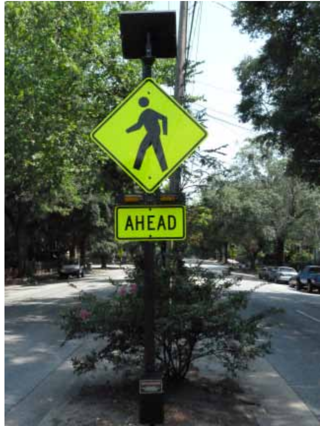
Example of Rectangular Rapid Flash Beacons (RRFB)
