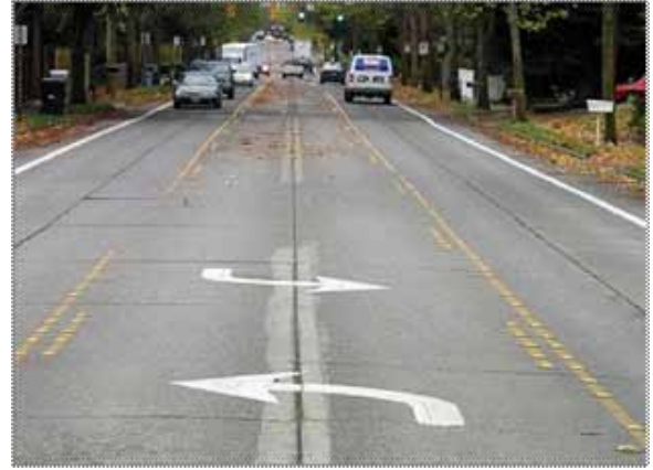
This road was re-striped to convert four vehicle travel lanes into three travel lanes with bike lanes.
