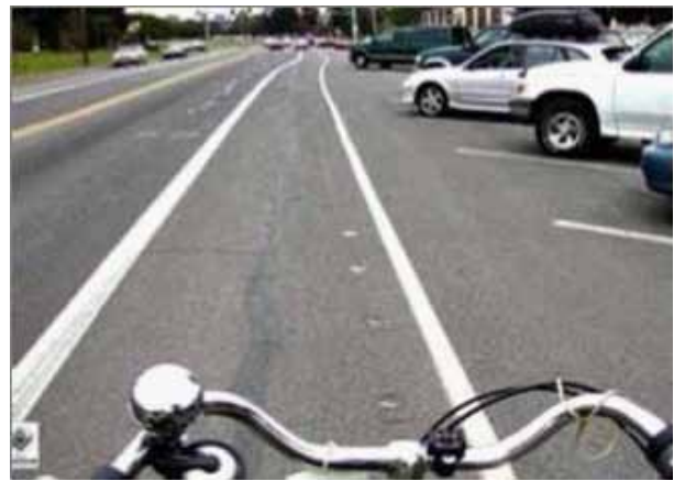
Back-in diagonal parking provides increased safety for bicyclists as compared to head-in diagonal parking due to drivers' improved visibility as they exit the parking spot
