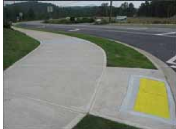
A diagonal curb ramp with detectable warning
