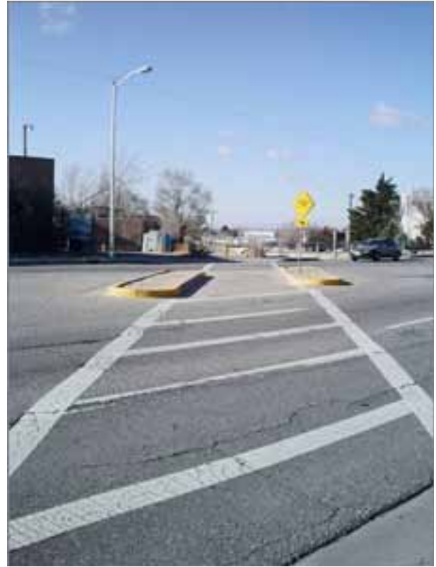
Ladder / zebra style crosswalks increase the visibility of pedestrians to drivers because the striping is in the same direction as the motorist path of travel.
