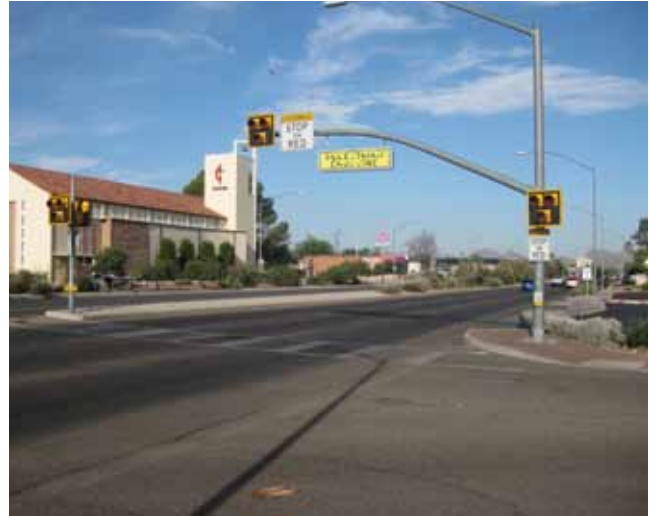
A hybrid beacon consists of a signal-head with two red lenses over a single yellow lens on the major street
