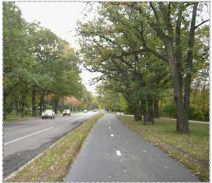
Trails directly adjacent to roadways can be challenging for users at roadway intersections.
