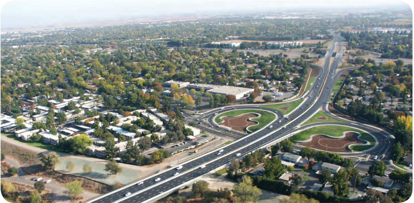
Watt Avenue Improvement Project improved mobility, safety, and seismic response for what had been one of the area's most congested roadways. The bridge was improved for motorists, cyclists, pedestrians, and residents. (Photo: SACDOT)
