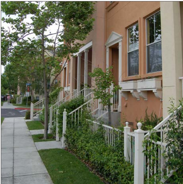
Setbacks provide buffering and transition to high density (top) and lower density (above) residential.
