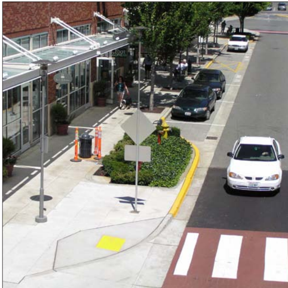
Corner bulbouts reduce the intersection crossing distance for pedestrians and provide additional streetscape amenity opportunities within the pedestrian zone.
