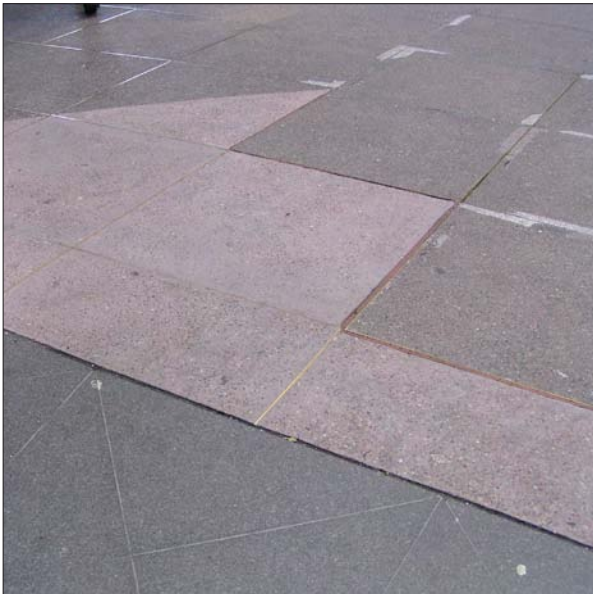
Special paving of public sidewalks should be avoided: it is difficult to maintain and repair with matching effects.
