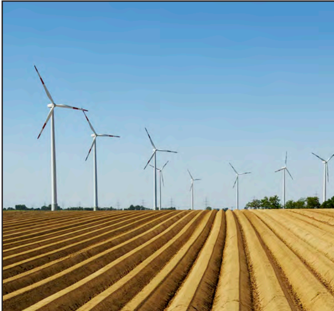
Horizontal-axis wind turbines are considered to be the best available technology for large-scale generation.
