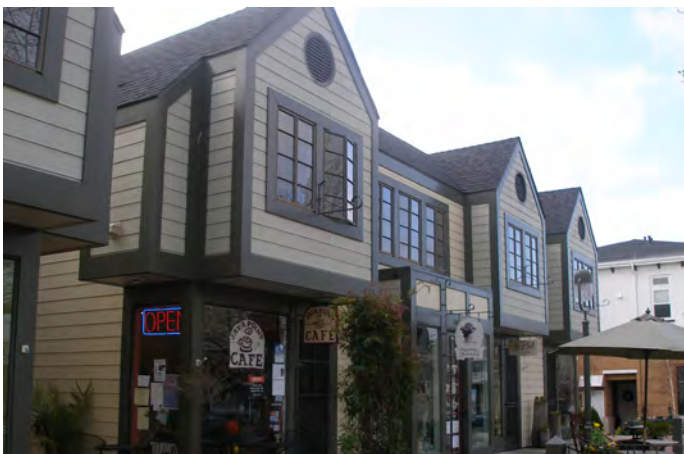
Mixed-use office and retail in the downtown (2008).
