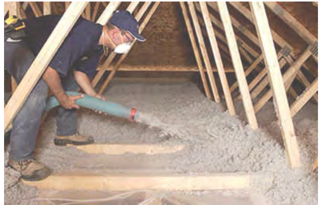
About 75% of El Cerrito homes are not adequately insulated. By properly sealing and insulating just the attic, homeowners could cut natural gas use by as much as 30%.
