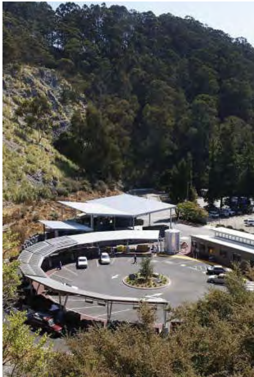
The new Recycling + Environmental Resource Center is EL Cerrito’s first LEED Platinum facility. Green building features include zero-net energy use, rain water catchment, rain gardens, and a Bay-Friendly native plantings.
